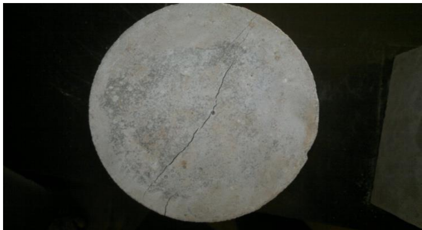
Fig -6: Crack developed along the Cross Section
