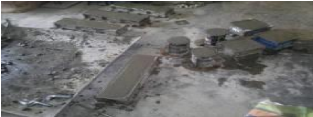
Fig -2: Casting under progress.
